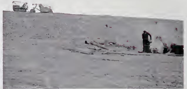
Bonneau Dam under construction
